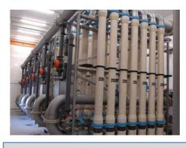
Fig. 5: Siemens' MemPulse™ MBR – a commercial installation.
