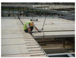
Fig. 1. Precast concrete hollow core slab placed onto steel beams.
