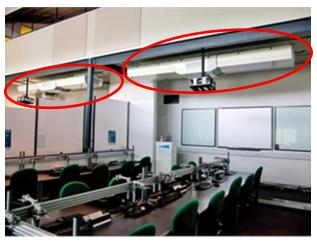
Figure 2: Two Cool-Phase units mounted on the ceiling of an ICT suite in the University of East London
